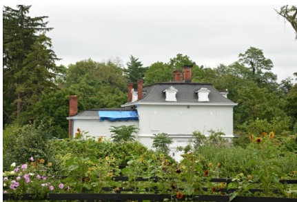
Blind House 35, Newburgh, NY
