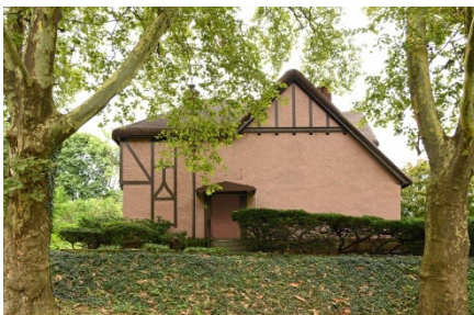
Blind House 30, Newburgh, NY
